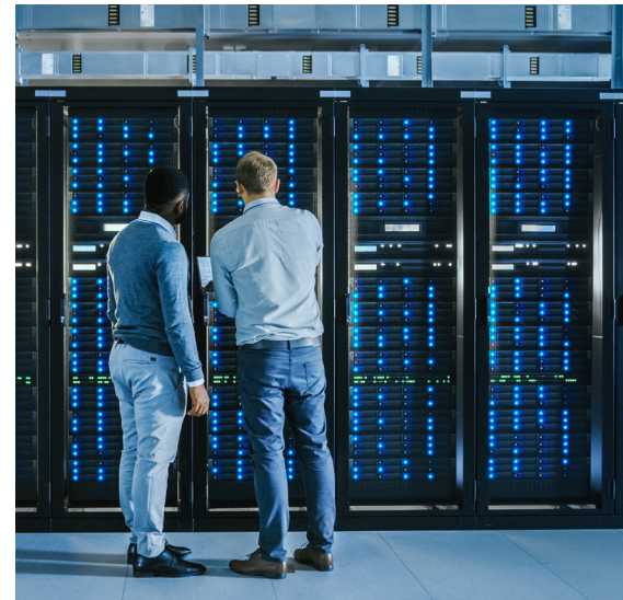
The secure transfer of data is critical to the business of an international fashion retailer in many ways. Dedicated Fiber Internet (DFI) service from Spectrum Business helps ensure information gets shared securely and without delay.
