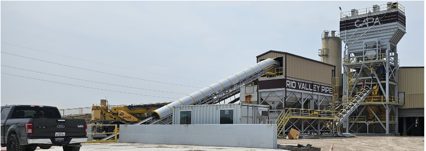
CAPA plants need to be able to run continually, without disruption. Helping them do just that is a Service Level Agreement (SLA) with Spectrum Enterprise guaranteeing 100% uptime.
