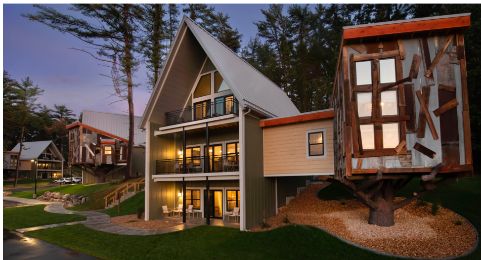
Secluded cabins offer guests a private place from which to enjoy the natural splendor of Wilderness Resort. They also presented a WiFi coverage challenge. Spectrum Enterprise solved it with Managed WiFi and strategically locating over 1,300 access points around the 600-acre property.
