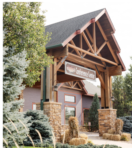
Business conferences are becoming a bigger part of business for Wilderness Resort. Having robust bandwidth available on site is critical to keep them coming back.
